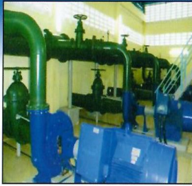
MABAYANI PUMPING STATION
